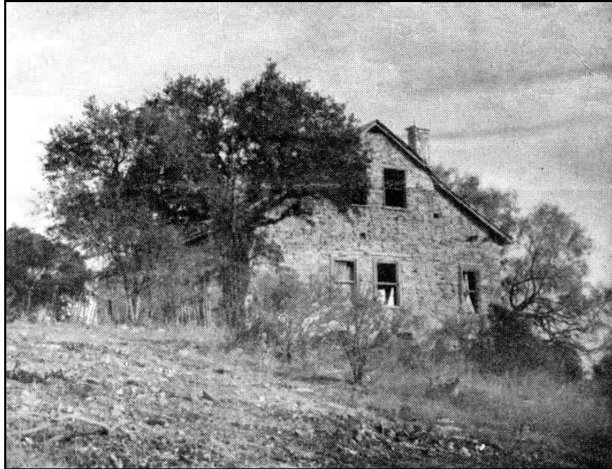
THE FUCHS PLACE — Here a century ago Adolph Fuchs established his family in what became the southern part of Burnet and Llano Counties, in the area of what today is becoming the Horseshoe Bay resort development. Developers of the Bay are clearing away cedar and brush preparatory for restoring the Fuchs home. The home is on land that is not part of Section One of Horseshoe Bay but has been acquired by the Bay's developers.
