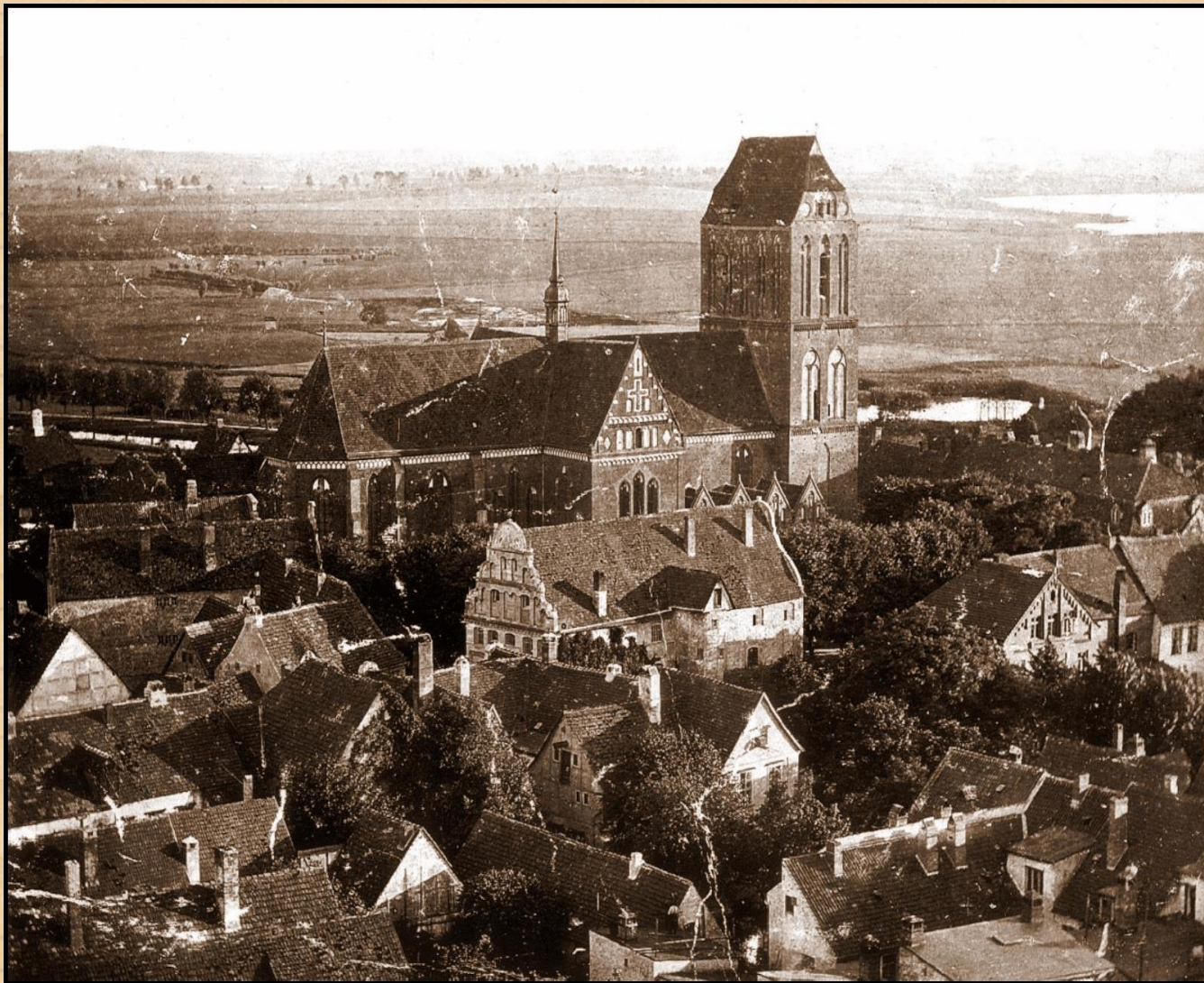
A view of Güstrow circa 1880. The Domschule can be seen in the center of the picture.
